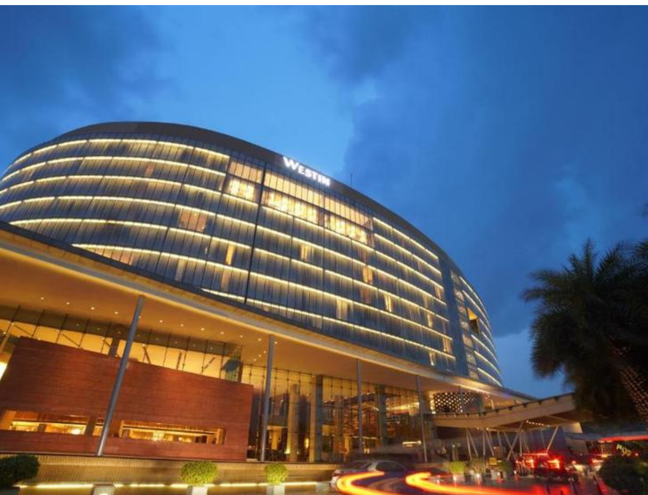
The Westin Gurgaon
